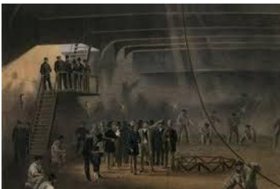
Caption: Cable coiled in the tanks of the SS Great Eastern
